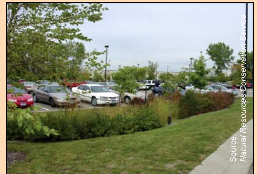
Parking lot incorporating bioretention area
