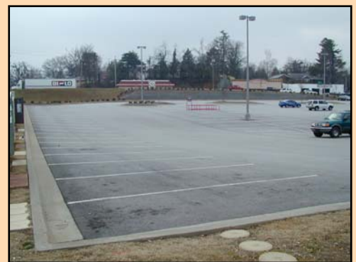
Parking lot lacking bioretention areas
