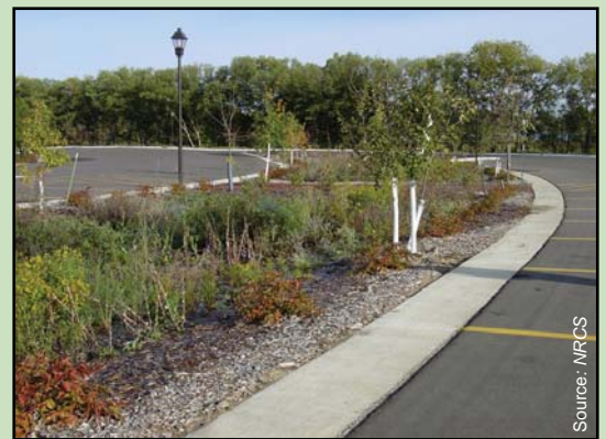
Parking Lot Bioretention Area Iowa
