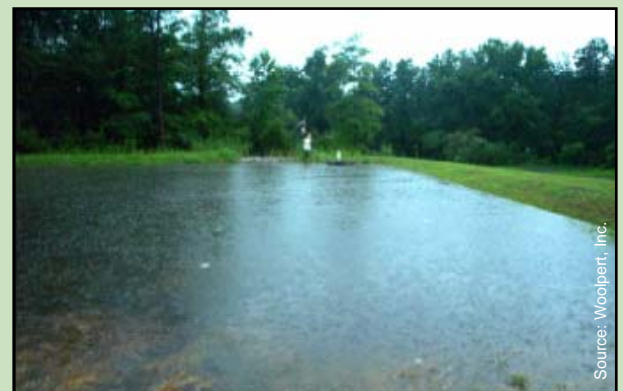
Our Lady of the Rosary bioretention area after storm event
