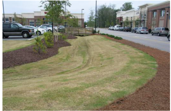
Wilmington, NC: Landscaped area in a mixed-use center that also serves as a storm water bio-retention catchment area.
