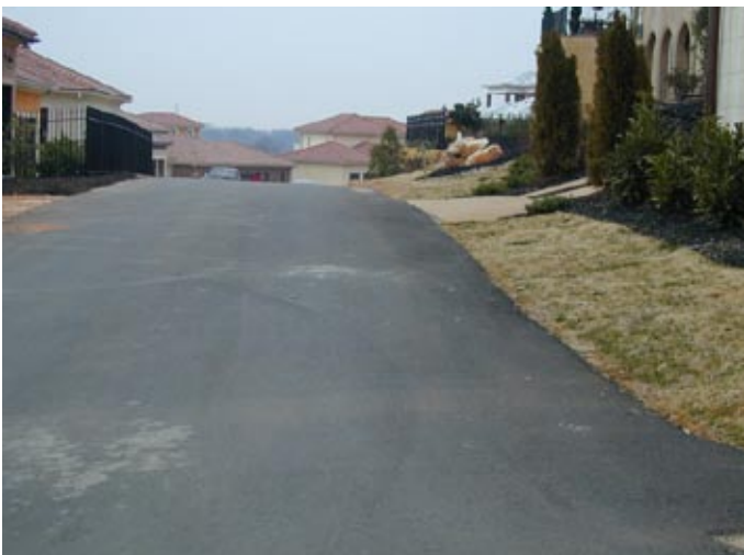
Greenville, SC: An approximately 20-foot wide alley in the Montebello development – again, substantially wider than necessary.
