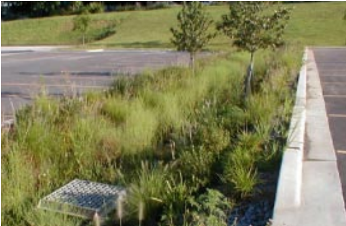
Washington, DC: A bio-retention parking lot median. Note the notches in the curb that allow sheet flow run off to enter the retention area.
