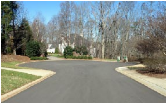
Greenville County, SC: On a cul-de-sac street, pavement could be narrowed by 2 to 4 feet given low volumes and low on-street parking.
