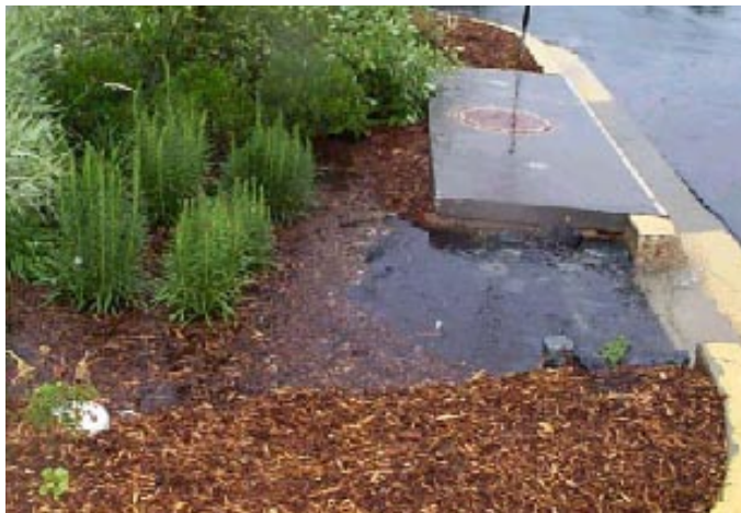
Landover, MD: A parking lot landscape island that was retrofitted as a rain garden. Note the area of the curbing that has been cut to allow sheet flow into the landscaped area.
