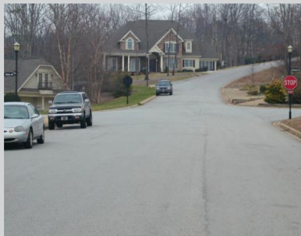
Greenville, SC: This street from the Montebello development is approximately 40 feet wide in the foreground, although it narrows to less than 30 feet as it goes up the hill. The amount of unused pavement in this example is quite dramatic, representing a missed cost saving opportunity for the developer of at least 8 to 10 feet for the widest section.
