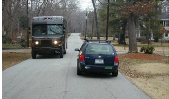
Greenville, SC: Grassed swale in an older large-lot neighborhood. The gentle slope of the swale on the right side of the street makes for an easily maintained area that can be mowed.
