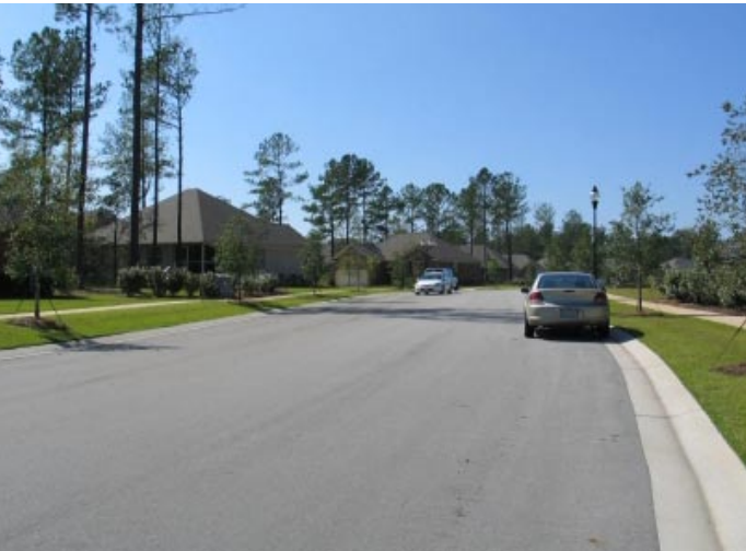
Leland, NC: This collector street has infrequent on-street parking, too much pavement (34 feet plus) – and, consequently, a speeding problem.
