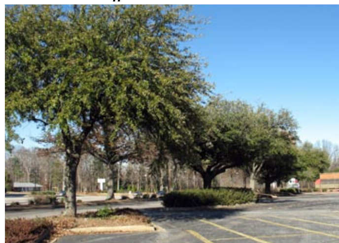
Greenville County, SC: While the landscaping in this lot provides some benefit, the curbed islands result in limited stormwater retention potential.
