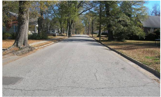
An approximately 24-foot wide street accommodates occasional parking on both sides (Clinton, SC). Source: Upstate Forever
