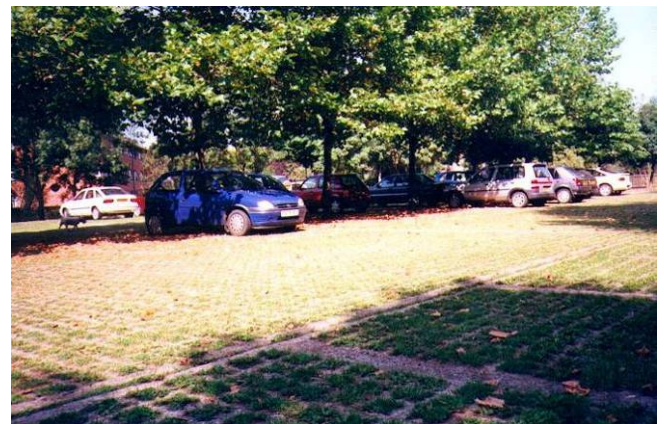
A parking lot with Grasscrete™ Interlocking pavers. Bordered by a stream and with no option for piped drainage, this parking lot has been draining naturally for 20 years (location unknown). Source: Bomanite Corporation
