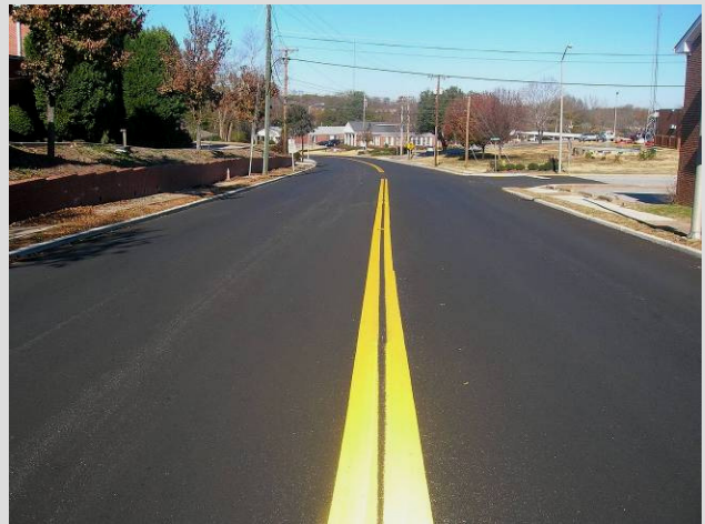
An example of a street that is approximately 40 feet wide. The amount of unused pavement represents a missed cost savings opportunity for the developer of at least 8 to 10 feet (Laurens, SC). Source: Upstate Forever
