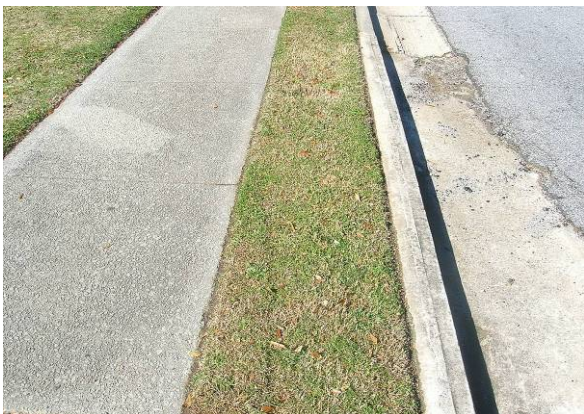
A two-foot planting strip provides little buffer from the street and is barely wide enough for grass, much less street trees (Westminster, SC). Source: UF
