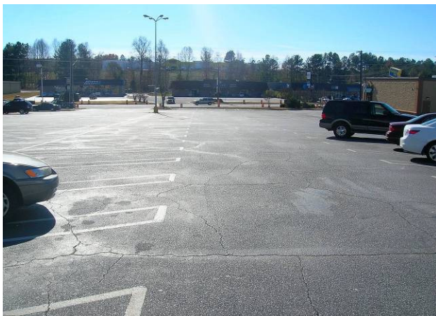
Parking lots and streets are one of the largest sources of impervious cover in urbanized areas (Laurens, SC). Source: Upstate Forever
