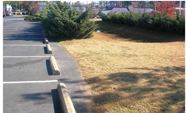
A bio-retention area used in a parking lot. Note the curbless edges that allow sheet flow runoff to enter the retention area (Laurens, SC) Source: UF
