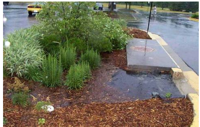
Parking lot landscape island retrofitted as a rain garden. Note curbing that has been cut to allow sheet flow into the landscaped area (Landover, MD). Source: Unknown
