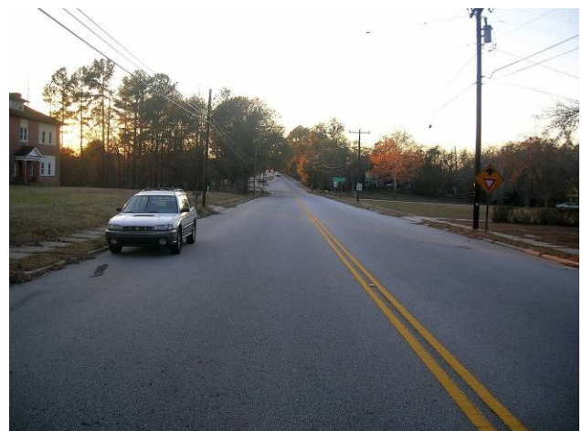
An example of a collector street that has infrequent on-street parking and unnecessary pavement, which likely encourages speeding (Hodges, SC). Source: Upstate Forever
