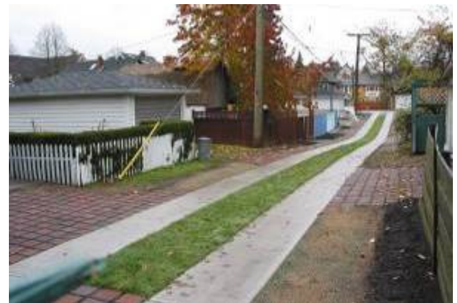
An alley with grass median and pervious parking pads (Vancouver, BC). Source: Puget Sound Action Team
