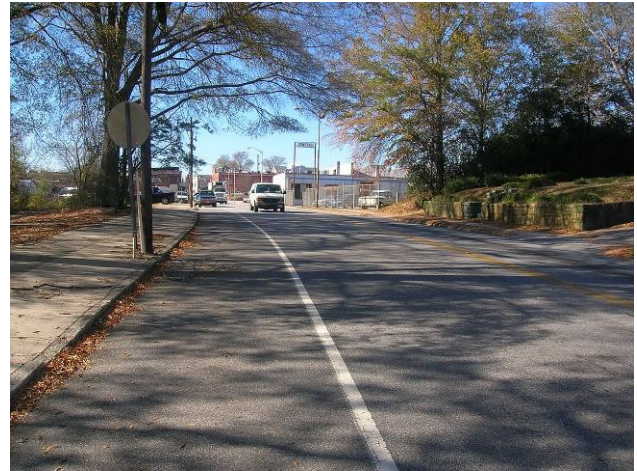
A 30 to 32-foot wide collector street with a parking shoulder (Laurens, SC). Source: Upstate Forever
