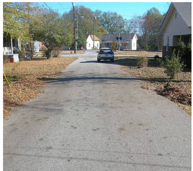
An example of a narrow street with no curb and gutter (Clinton, SC). Source: Upstate Forever
