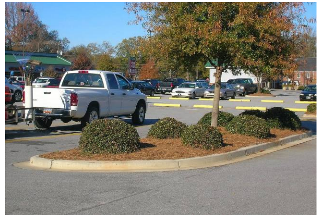
While increased parking lot landscaping provides many benefits, the curbed islands result in limited storm water retention potential (Greenwood County, SC). Source: Upstate Forever
