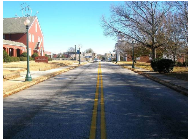
This 30 to 32-foot wide collector street may be appropriate given the regular on-street parking on Sundays (Laurens, SC). Source: The Lawrence Group
