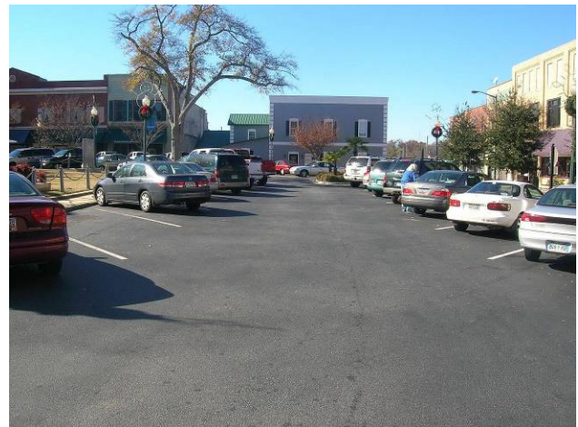
Narrow drive aisles in off-street parking lots decrease the costs of providing parking while minimizing the amount of pervious area (Laurens, SC). Source: Upstate Forever
