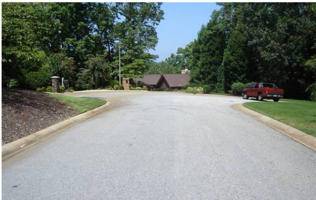
On this cul-de-sac street, pavement could easily be narrowed by 4 to 6 feet (Oconee County, SC). Source: Upstate Forever
