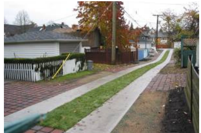
An alley with grass median and pervious parking pads (Vancouver, BC). Source: Puget Sound Action Team
