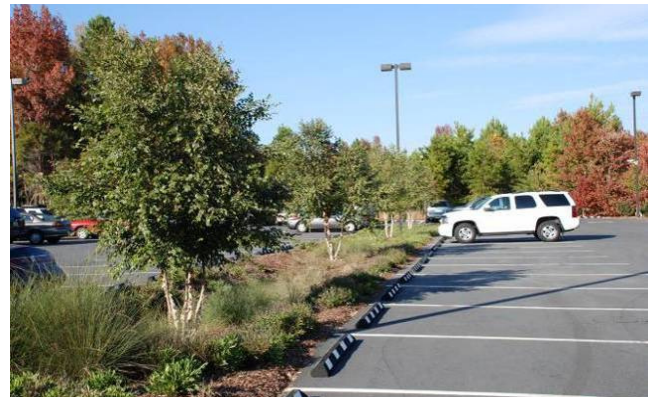
A bio-retention parking lot median. Note the curbless edges that allow sheet flow run off to enter the retention area (Huntersville, NC)
