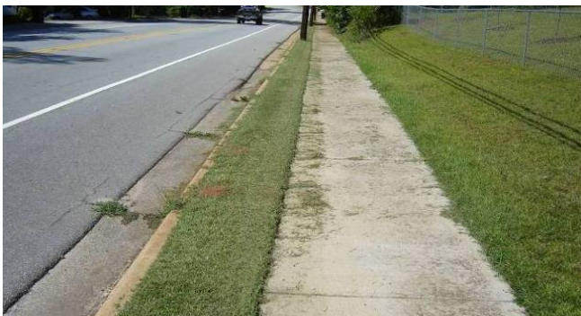
A two-foot planting strip along a sidewalk is barely wide enough for grass, much less street trees, and provides little buffer from the street (Westminster, SC). Source: Upstate Forever
