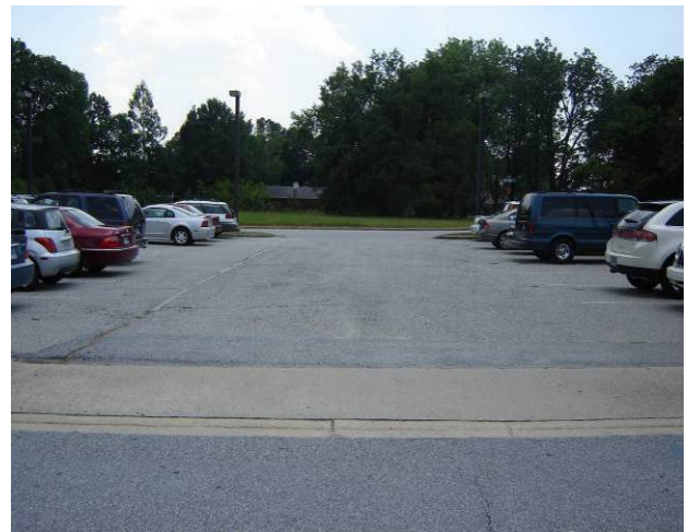
Overly large drive aisles in off-street parking lots increase the costs of providing parking and decrease the amount of pervious area (Walhalla, SC). Source: Upstate Forever
