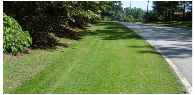
The gentle slope of the swale on the side of this street is an easily maintained area that can be mowed (Oconee County, SC). Source: Upstate Forever
