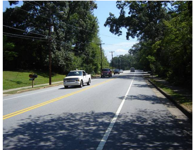
A 30 to 32-foot wide collector street with bike lanes (Westminster, SC). Source: Upstate Forever
