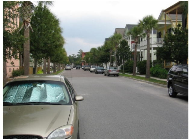
This 30 to 32-foot wide collector street may be appropriate given the frequent on-street parking (Mt. Pleasant, SC). Source: The Lawrence Group
