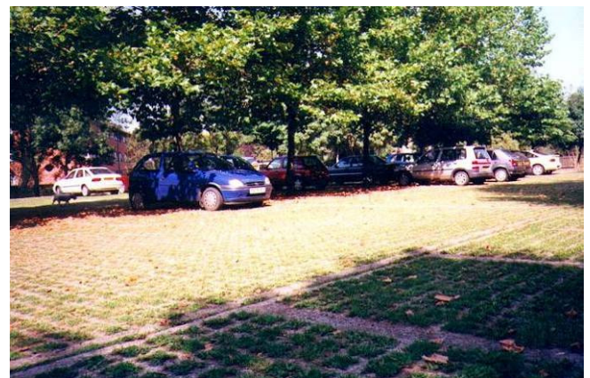
A parking lot with Grasscrete™ Interlocking pavers. Bordered by a stream and with no option for piped drainage, this parking lot has been draining naturally for 20 years (location unknown). Source: Bomanite Corporation
