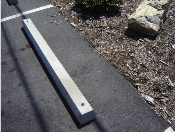
Parking area landscaping with no curbing allows for more effective infiltration of storm water when it is at grade or below (Salem, SC). Source: Upstate Forever
