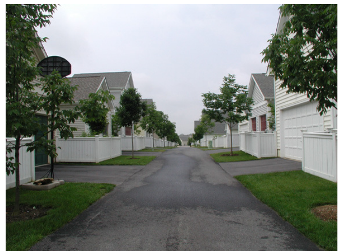
A 12-foot alley with trees and no curbs serves houses on approximately 40-foot wide lots (Gaithersburg, MD). Source: The Lawrence Group
