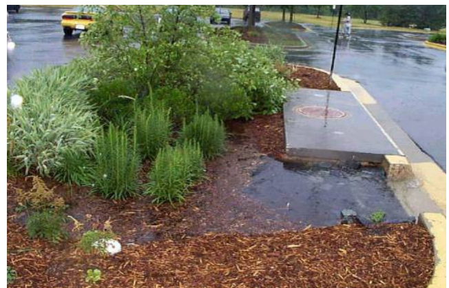
Parking lot landscape island retrofitted as a rain garden. Note curbing that has been cut to allow sheet flow into the landscaped area (Landover, MD). Source: Unknown
