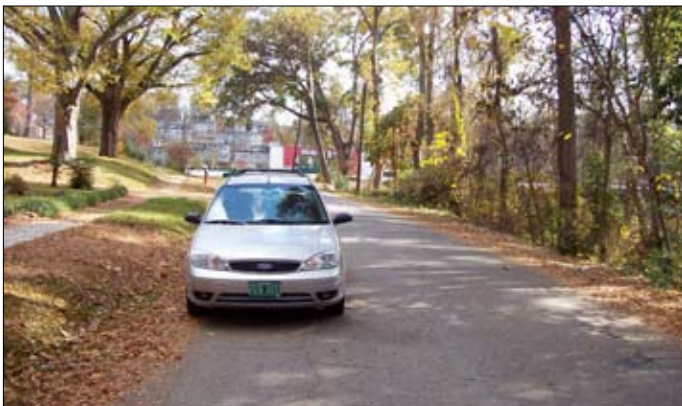
An example of a narrow street with no curb and gutter (Spartanburg County, SC).
