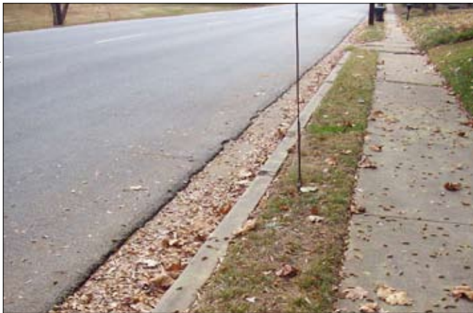
A two-foot planting strip along a sidewalk is barely wide enough for grass, much less street trees, and provides little buffer from the street (Anderson County, SC).
