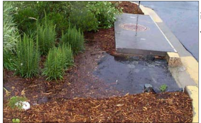
Parking lot landscape island retrofitted as a rain garden. Note curbing that has been cut to allow sheet flow into the landscaped area (Landover, MD).
