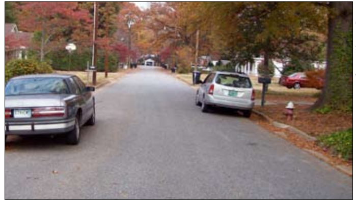
An approximately 24-foot wide street accommodates occasional parking on both sides (Anderson County, SC).
