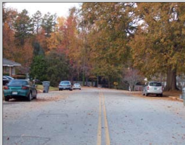
An example of a street that is approximately 40 feet wide. The amount of unused pavement represents a missed cost savings opportunity for the developer of at least 8 to 10 feet (Spartanburg County, SC).
