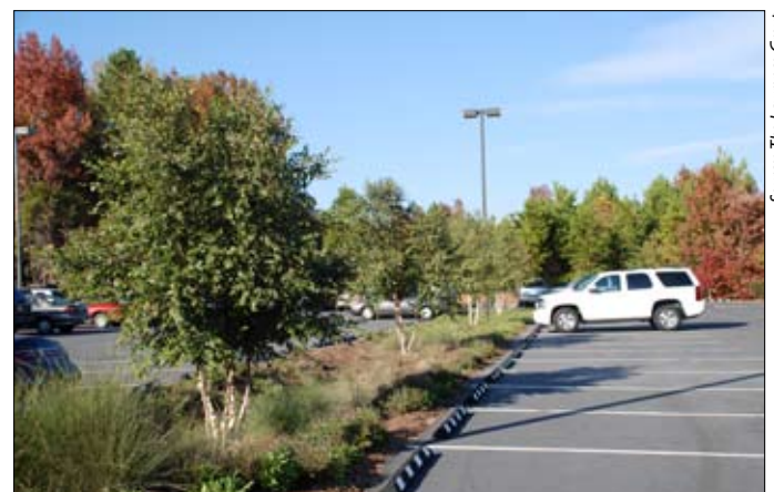
A bio-retention parking lot median. Note the curbless edges that allow sheet flow run off to enter the retention area (Huntersville, NC).
