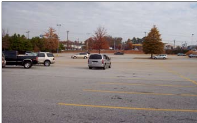
Limited landscaping as well as grading that slopes away from landscaped areas provides little opportunity for natural infiltration of stormwater (Anderson County, SC).
