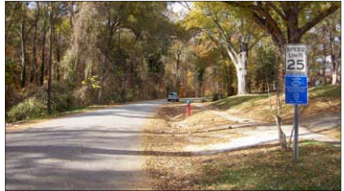
Grassed swale in an older, large-lot neighborhood. The gentle slope of the swale on the right side of the street makes for an easily maintained area that can be mowed (Spartanburg County, SC).
