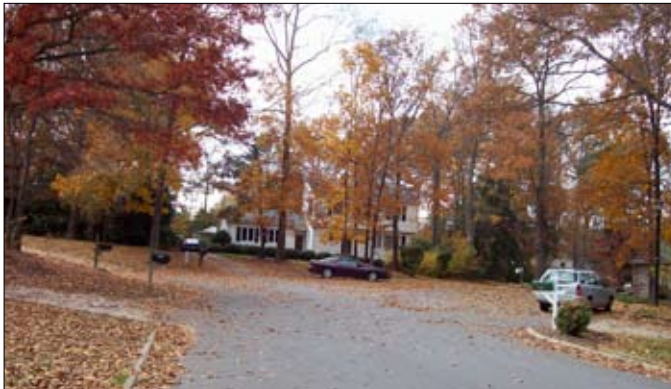
On this cul-de-sac street, pavement could easily be narrowed by 4 to 6 feet (Spartanburg County, SC).
