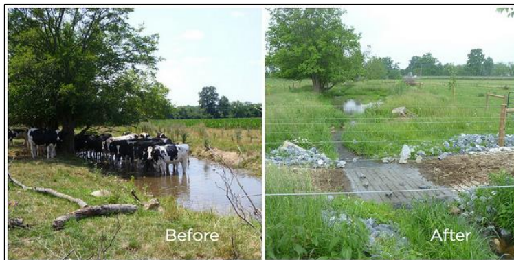
Example of Armored Streambank Crossing
